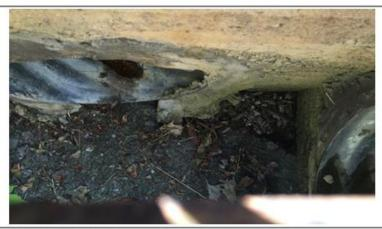
Photo 1: Sump needs to be cleaned out.
