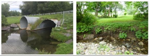
Photo 1: Culvert carrying Sucker Brook beneath VTRoute 30. Photo 1: Sucker Brook bank erosion along the north bank approximately 200ft upstream of Route 30 crossing Project Type: Stream Channel/Bank Erosion, Prioritization by project type: High
