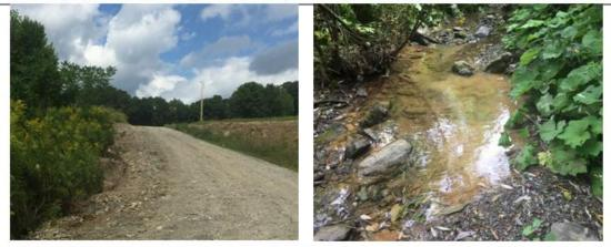
Photo 1: Erosion from driveway, cleared area, and ditch drains to Sucker Brook. Photo2: Evidence of driveway sediment is seen in the brook near the bridge.
