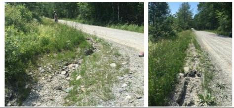
**Photo 1:** Erosion and road runoff runs to Sucker Brook. Photo from top of culvert **Photo 2:** Road ditch has grown in with vegetation and is not connected to the road, causing eroding along the length of the road. The road ditch can be reshaped and stabilized with rock and/ or check dams.
