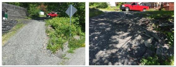
Photo 1: Steep driveway drains to Lake Road and the lake. Existing catch basin located behind road sign. Photo 2: Close up of the most eroded area on the driveway.
